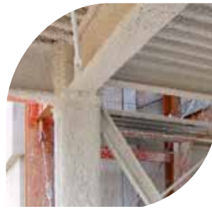
ST. THERESA VILLA BAGHERIA (PA) ITALY
