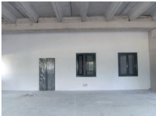
LODI: dividing walls for offices and canteen.
